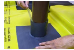
Slide the top hat into position and push down on the flat section to effect a seal on to the tape. Carefully remove the plastic release membrane from the tape around the pipe by pulling it out.
