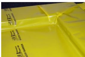
It is possible to complete internal corners by using a "hospital fold" method. Ensure voiding behind membrane is minimal
