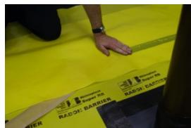
Remove the release paper and apply pressure to effect a seal. Expel any air trapped in the gasket. A roller is useful for this purpose
