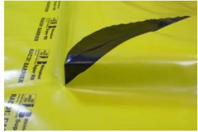
Tuck the membrane neatly into the floor/wall angle to prevent excess voiding behind.
