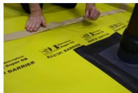
Overlap the Gas Barrier to a minimum of 150mm. Place a strip of Rhinoplast LT Jointstrip on the lower layer, having removed the plastic release film from the tape and press down firmly.
