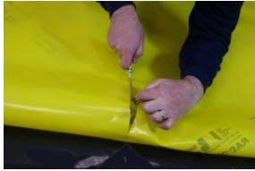
A preformed cloak is required for external corners. Cut the membrane at 45 degrees from the corner to release tension and achieve a neat fit.
