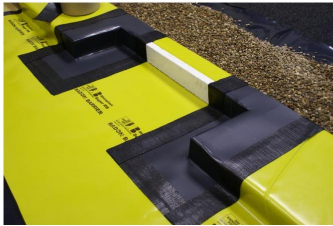
Where door thresholds are necessary, a preformed cloak pair is available which should be installed using the sealing and detailing method described for the corners.
