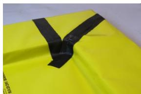
Secure corners to hold in place with Rhinoplast Reinforced Detail Strip.
