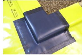
Remove the brown release paper on the Jointstrip and push the cloak onto the tape to effect a seal. Over - tape with Rhinoplast Reinforced Detail Strip.
