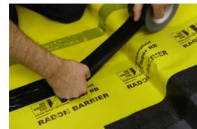
Secure the flap down with Rhinoplast High Tack single sided girth tape to secure the joint and protect it from the concrete pour.
