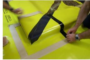
Place strips of Rhinoplast LT Jointstrip under the footprint of the cloak ensuring corners are butt jointed.
