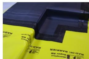
For ease of installation, internal corner cloaks are available. All preformed cloaks should be sealed with Rhinoplast LT Jointstrip and over-taped with Rhinoplast Reinforced Detail Strip.
