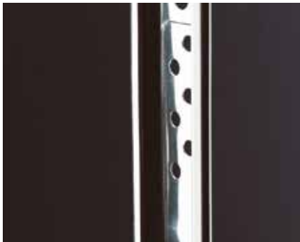
SWS (detail of tie folded up into channel)
